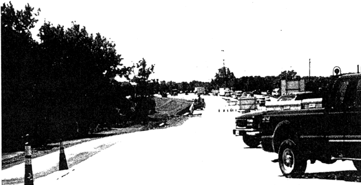
Part of the finished product is almost ready for traffic. This is the first of four phases that will be completed in two years. The slip formed concrete pavement is designed for 50-year usage.
