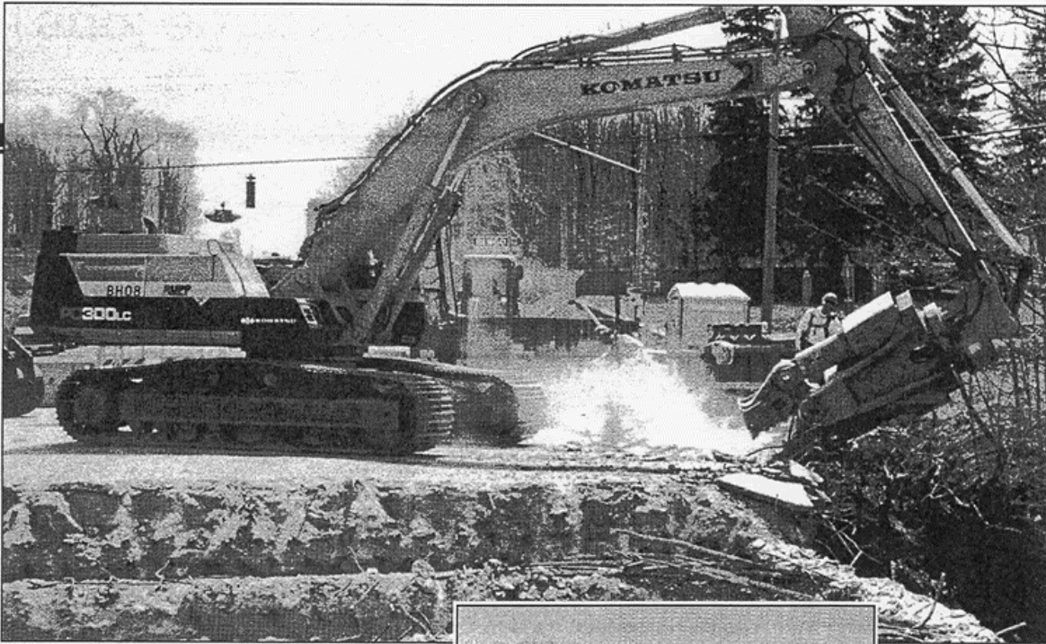
A Komatsu PC300LC excavator with LaBounty UP50 Universal Processor is being used to demolish a bridge deck on the Route 20 bridge over Eighteen Mile Creek Road in the town of Hamburg.
